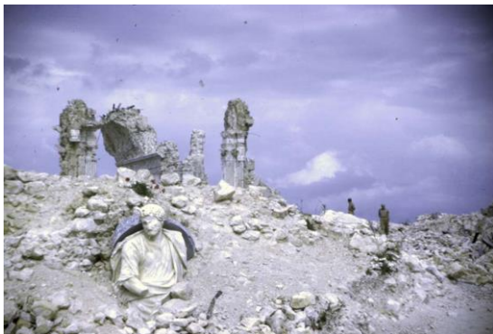
Figure 44: An image of Monte Cassino destroyed.
